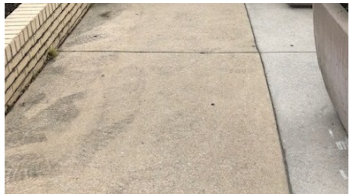
10th St photo after.
