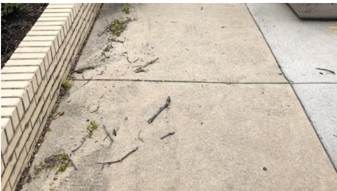
10th street sidewalk before.
