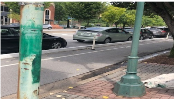
Before photo of light pole painted on Broad Street.
