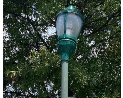
Ambassador noticed leaning light fixture and reported to EPB.
