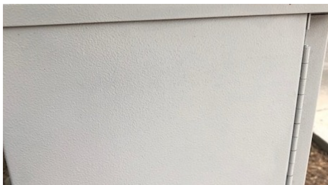
After photo of graffiti removed off electrical box.
