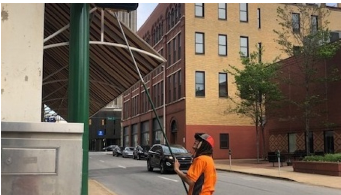
Ambassador Carson paints a pole on 7th St.
