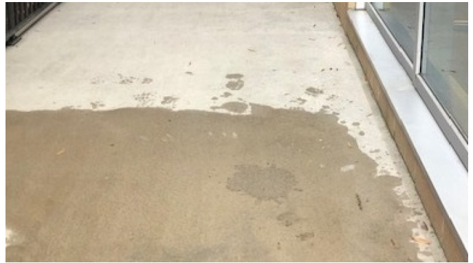
Biohazard removed from Broad St sidewalk.
