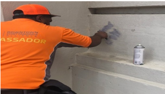
Ambassador Emanuel removes graffiti at Market Street bridge.
