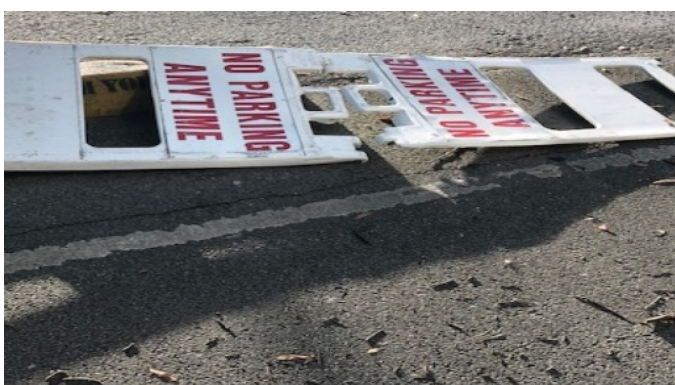
Fallen parking sign on Broad Street.
