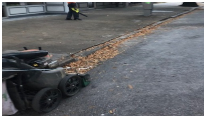
Before photos of curb line on Broad Street.
