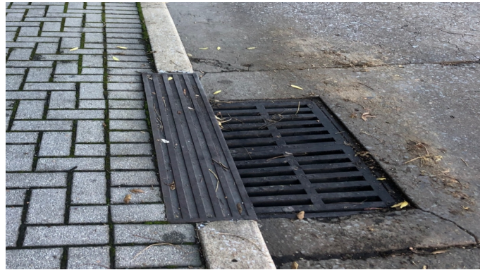
Catch basin 4th street after photo.
