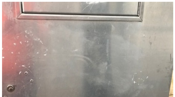
Graffiti removed from electrical box.
