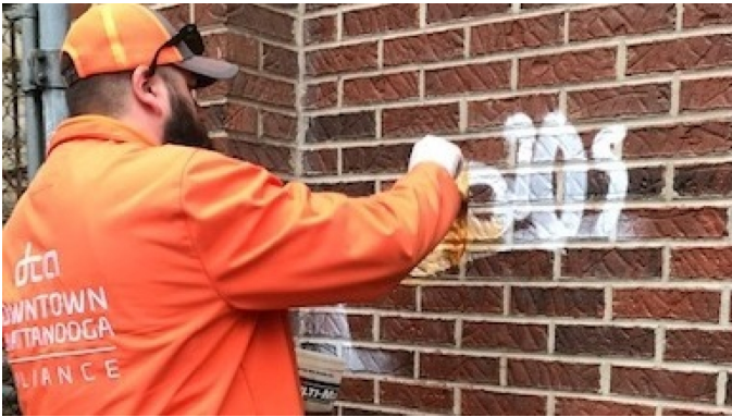
Team Leader Ryan applies graffiti remover to a building on Patten.
