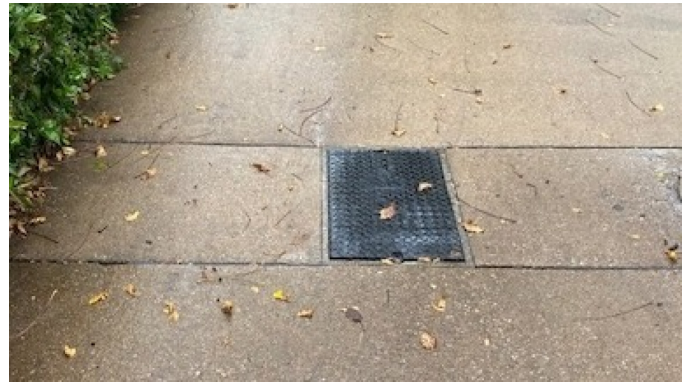
Sidewalk cover repaired on 3rd St.
