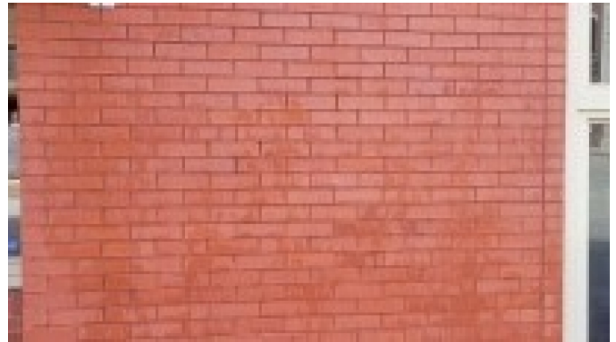
Graffiti tag removed from Cherry St building.
