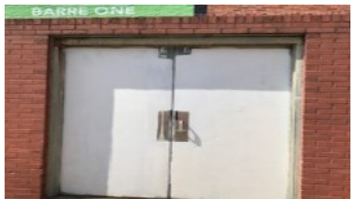
After photo of graffiti removed on Broad St.
