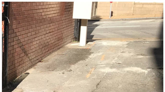
Alley off 7th St after clean-up.
