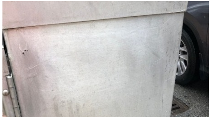
Graffiti removed from electrical box.
