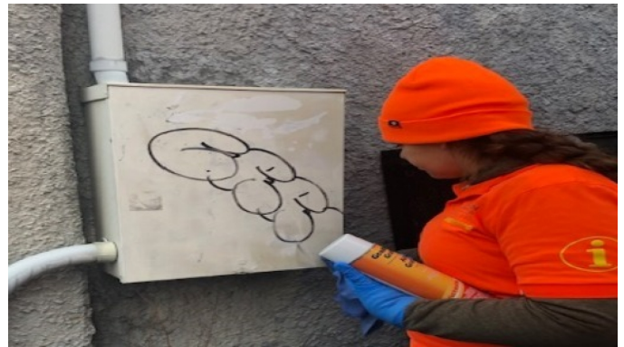
Kathy gets ready to remove graffiti on 8th St.
