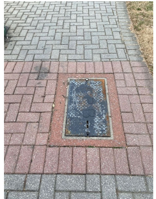
Cover on Chestnut repaired (less than 24hrs).
