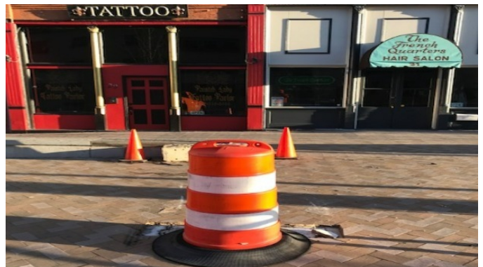
DCA puts out cones for pedestrian and vehicle safety.
