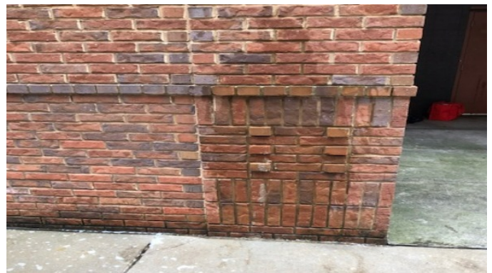
Biohazard on 3rd St after photo.
