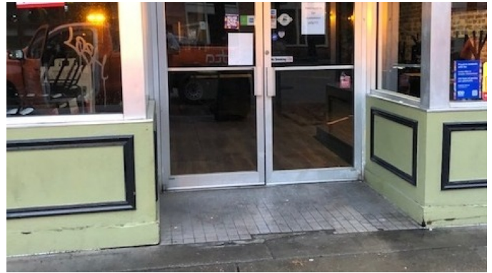
After photo of doorway cleaned up.
