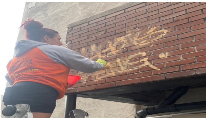
Randi applies graffiti remover on 7th Street.
