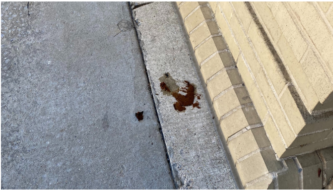
Biohazard on 10th Street.
