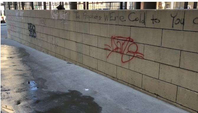
Parking garage wall Georgia St.
