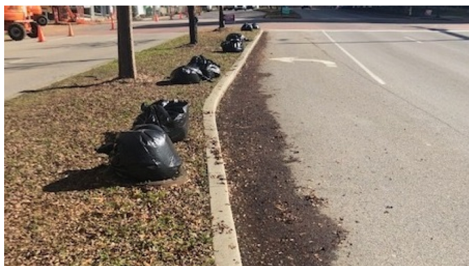
4th street center island after debris removed.
