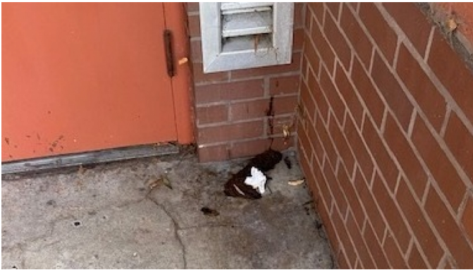
Biohazard in doorway at Loveman's Building.
