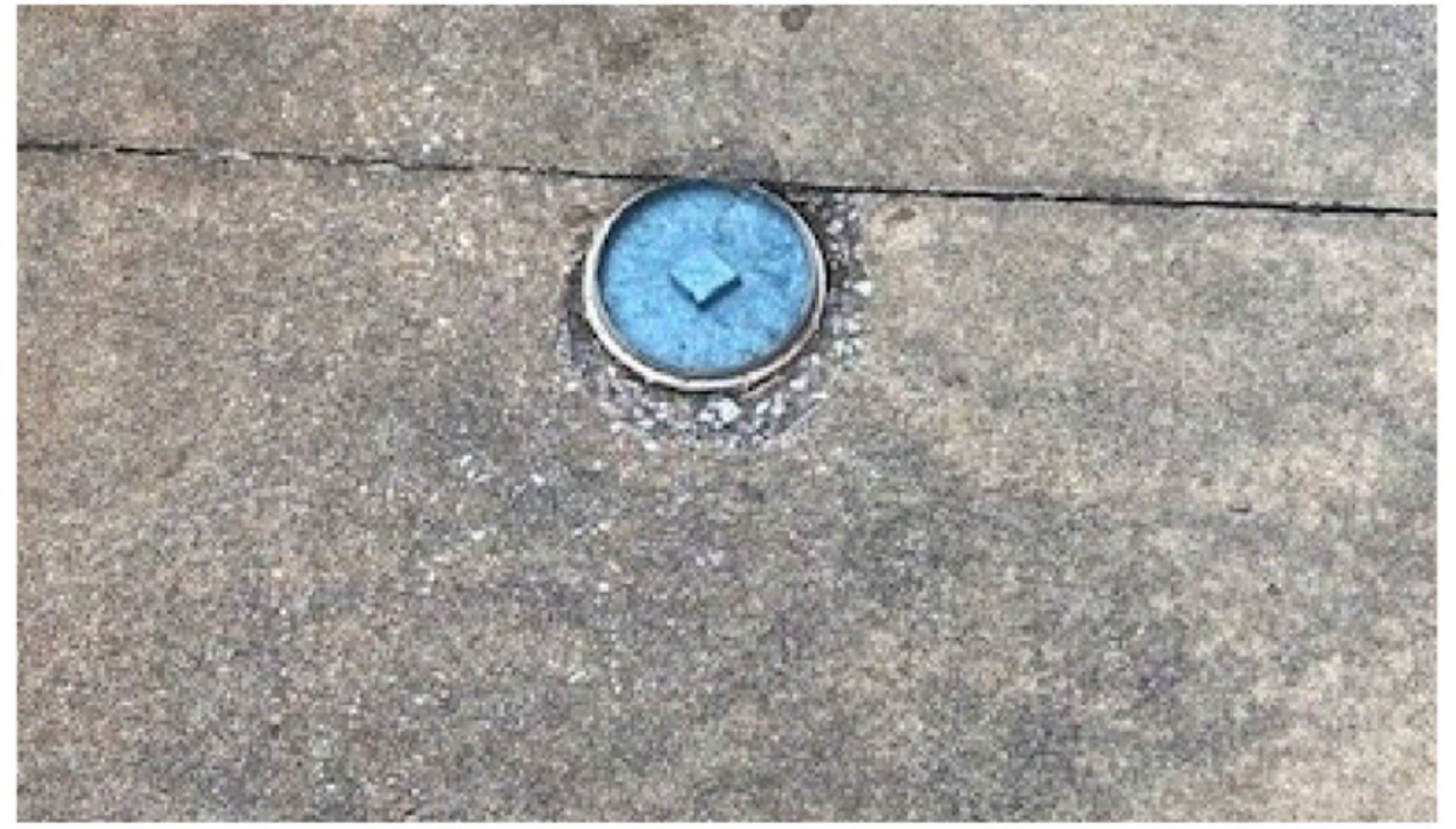
Cover placed back on Broad St sidewalk.
