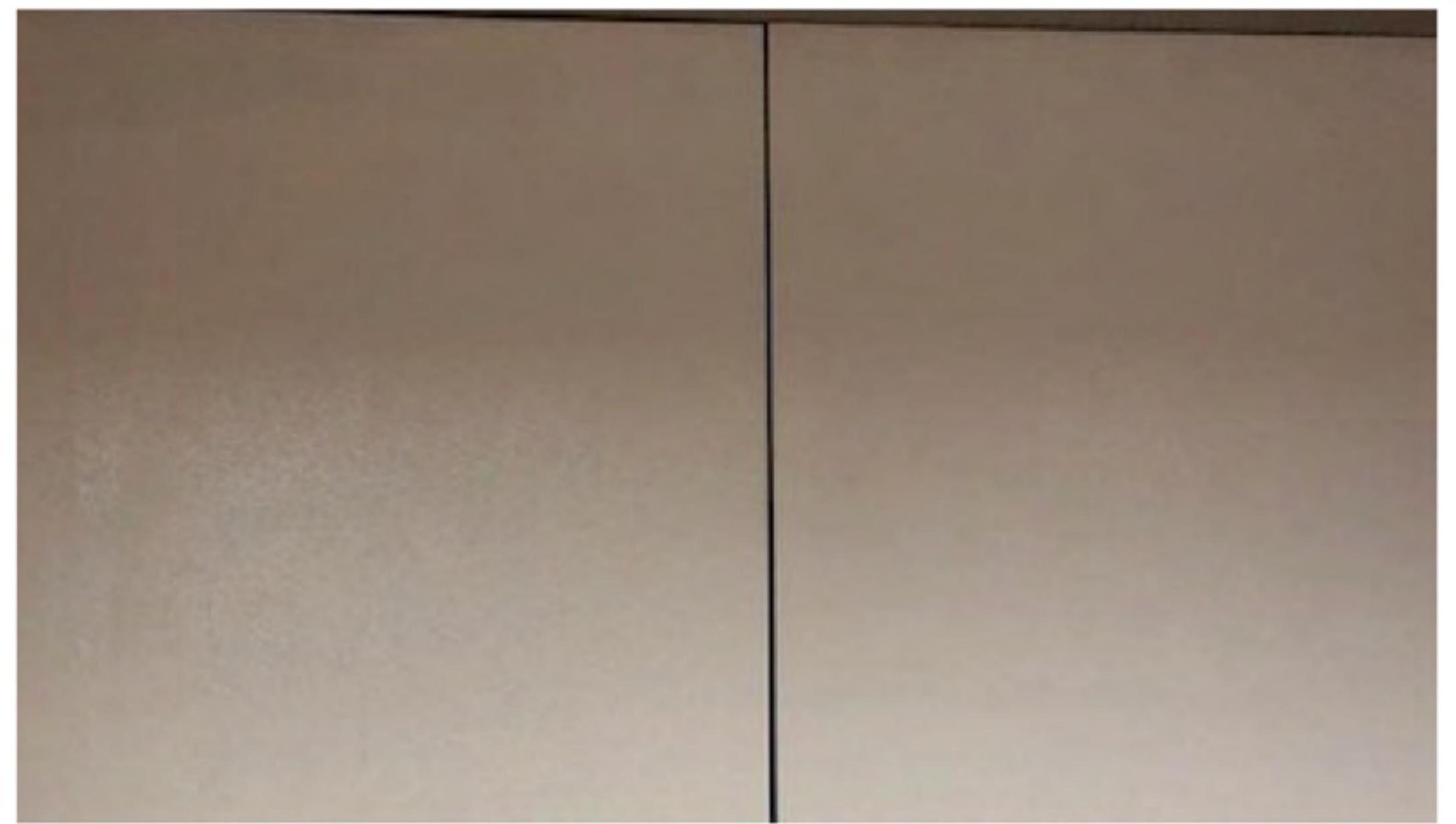
After photo of graffiti painted over on Chestnut St.
