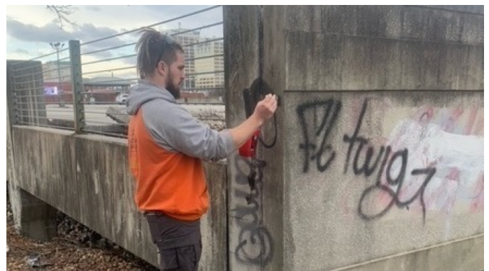
Team Leader Jake applies graffiti remover to garage on 3rd St.
