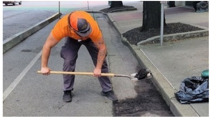
Ambassador Jake shovels dirt out of the curb line.
